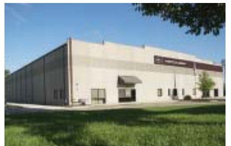
HIMOINSA POWER SYSTEMS INC.
